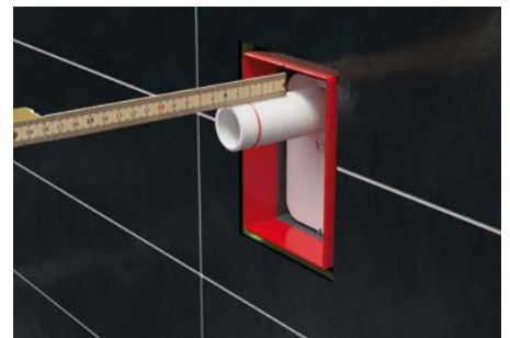
6. Mark 3cm, measured from the wall (tile)
